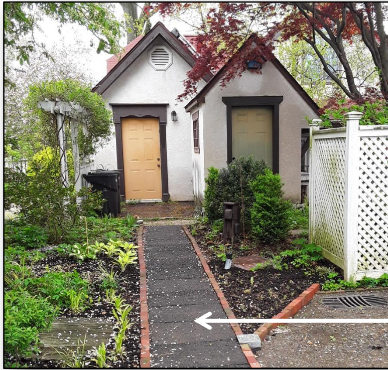
Asphalt pavers and salvaged brick edging
