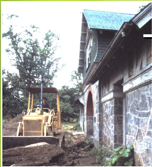
1986 Façade faces southwest
