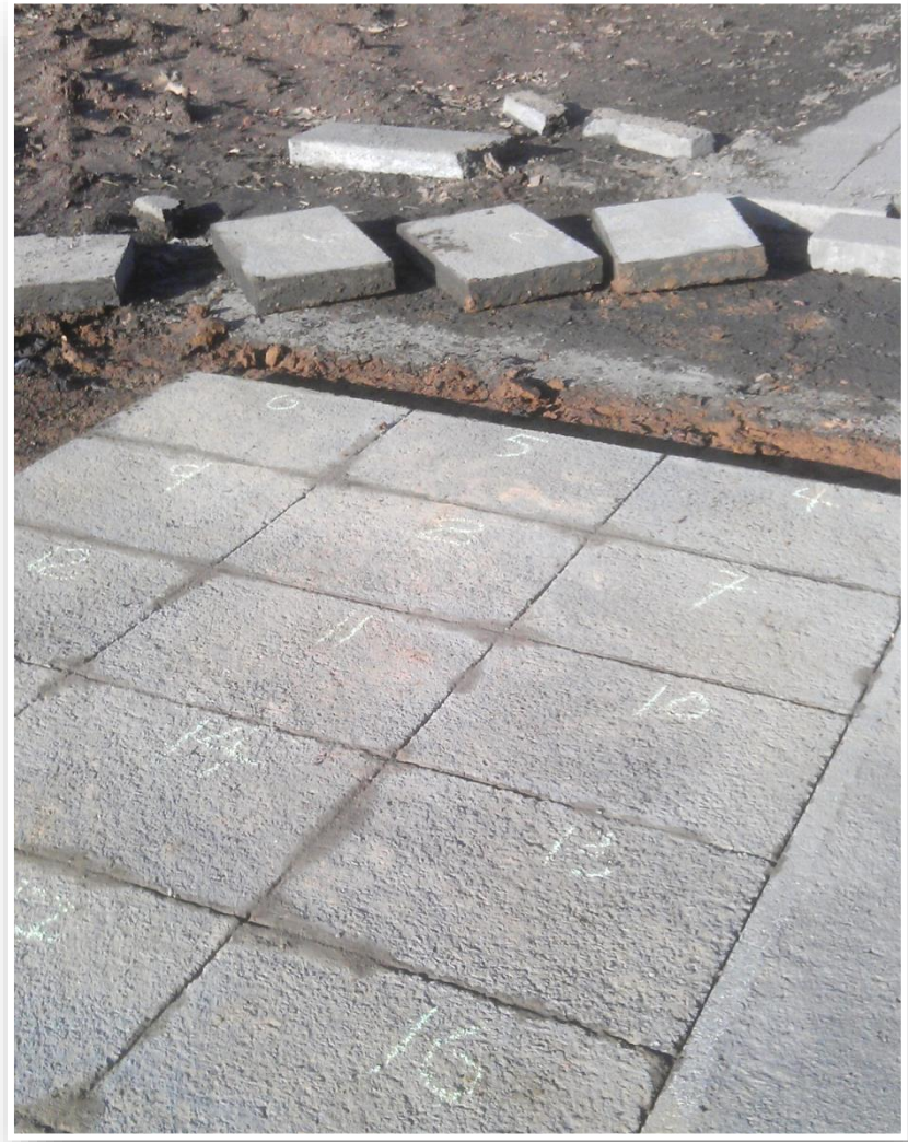
Asphalt tennis court cut for pavers
