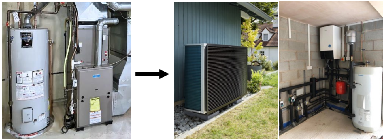
Gas furnace, A/C unit, and Gas Water Heater replacement ⇒ Whole home electrification
